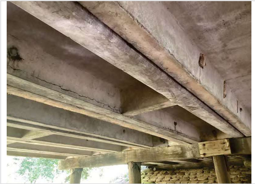
Span 2 bottom deck typical of all spans
